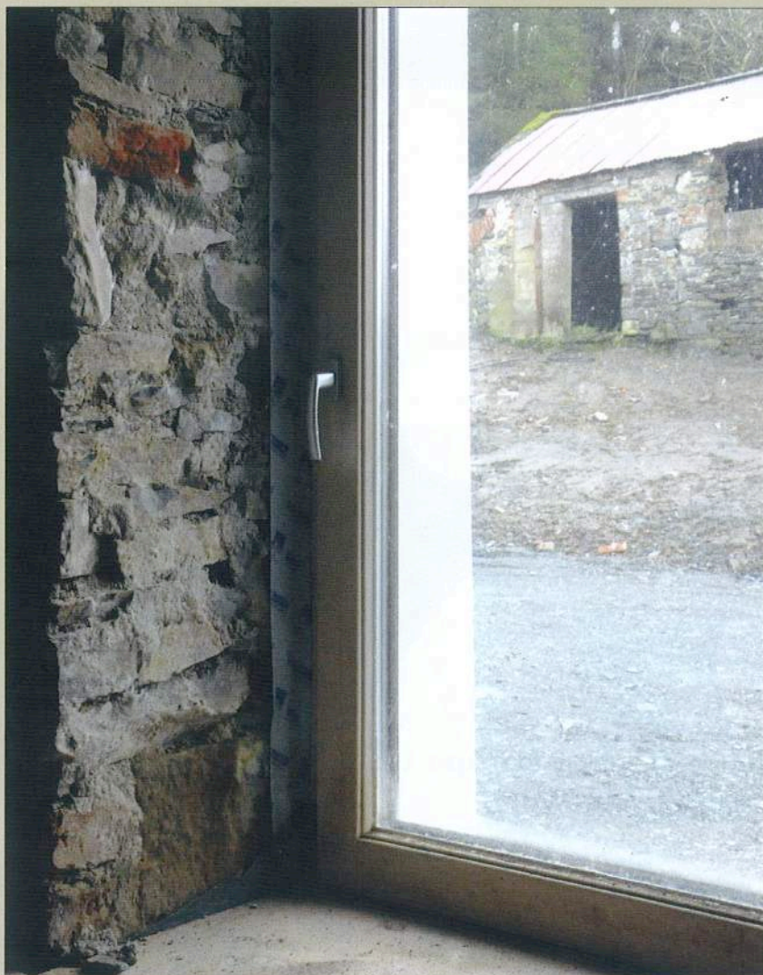
(p47) On the exterior of the house is a lime render, which improves the breathability of the building; (this page, above) The large stone walls of the house provide good thermal mass; (below) the house's windows are all triple-glazed units supplied by Optiwin
