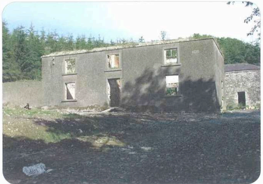
Original semi-derelict building
