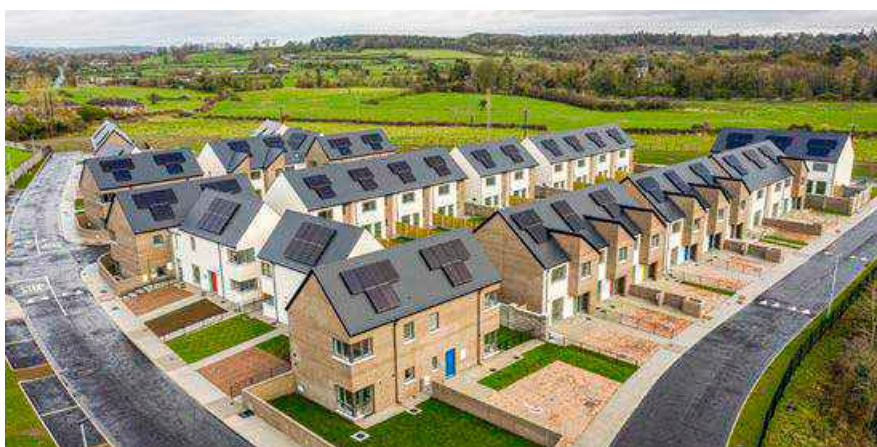
Local authority social housing forming a perimeter block with back to back gardens in the block centre. Riverside Kells, Cooney Architects.
